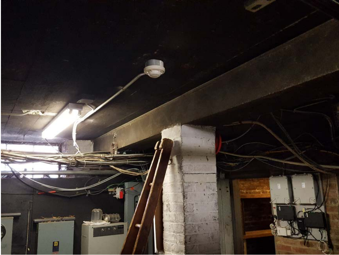
Photo #22 – Typical First Floor Concrete Construction above Basement.
