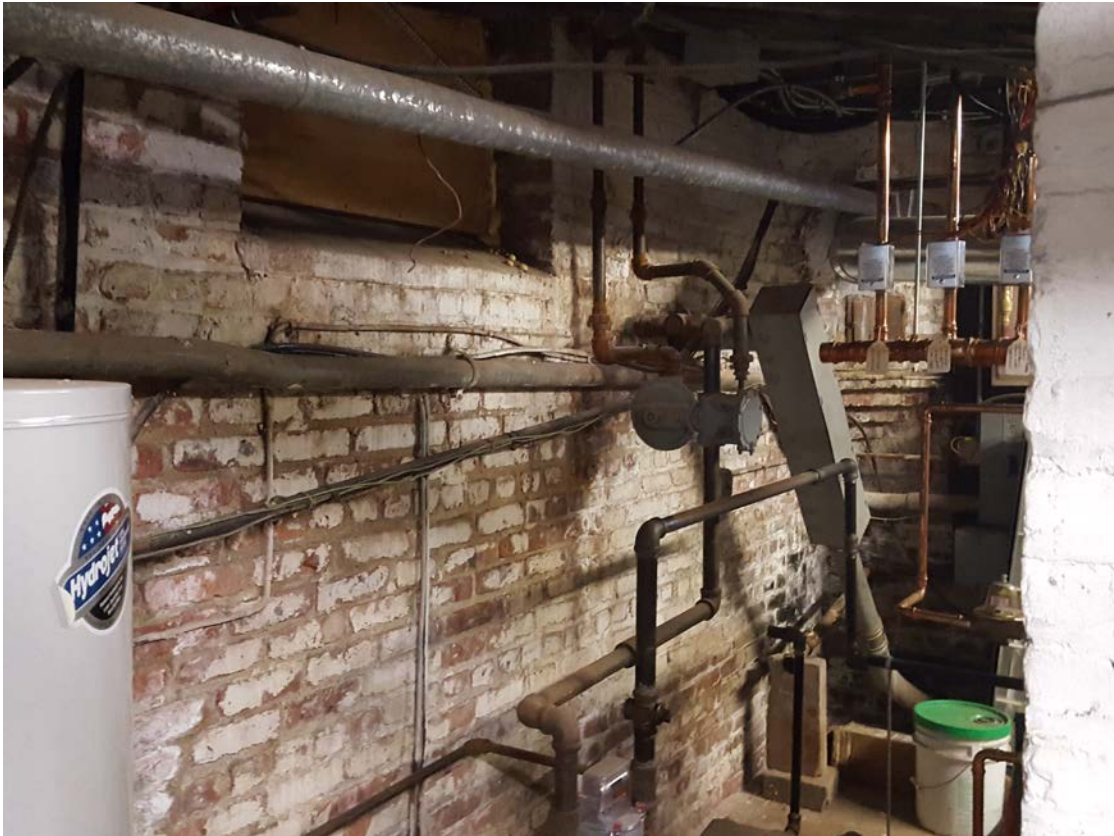
Photo #23 – Basement Wall Construction.
