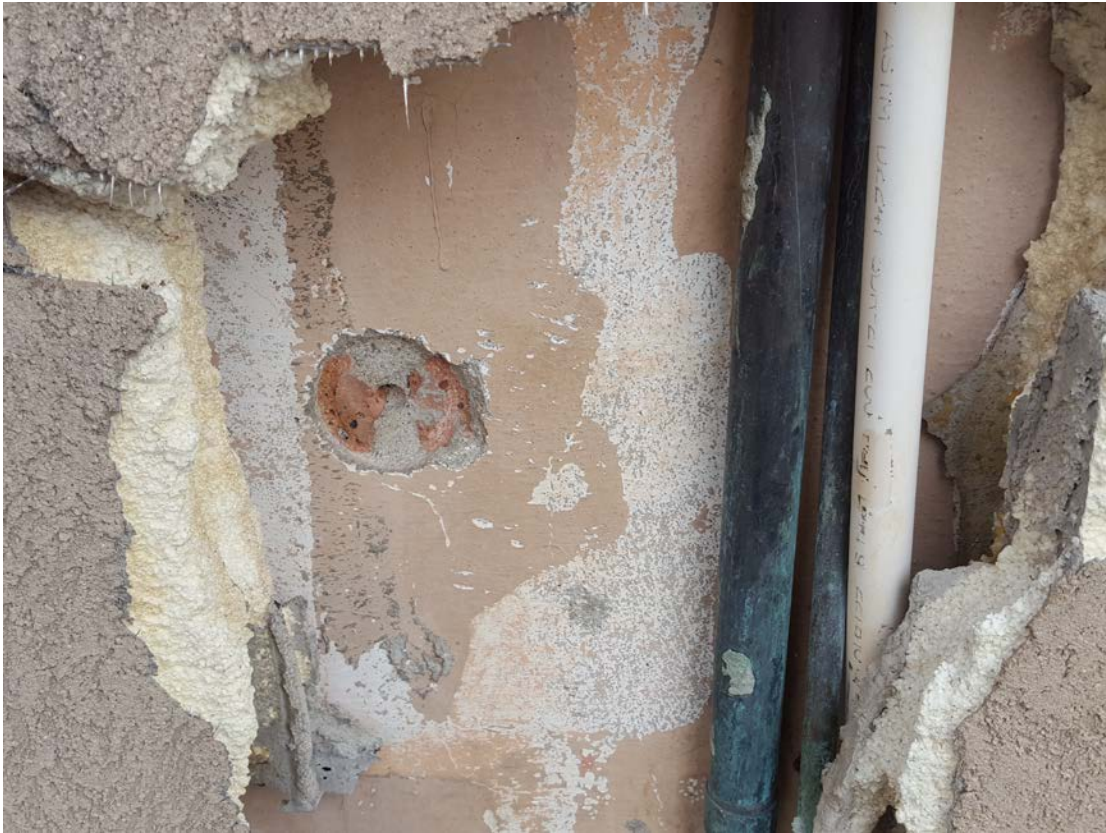
Photo #7 – Exterior Wall Construction.
