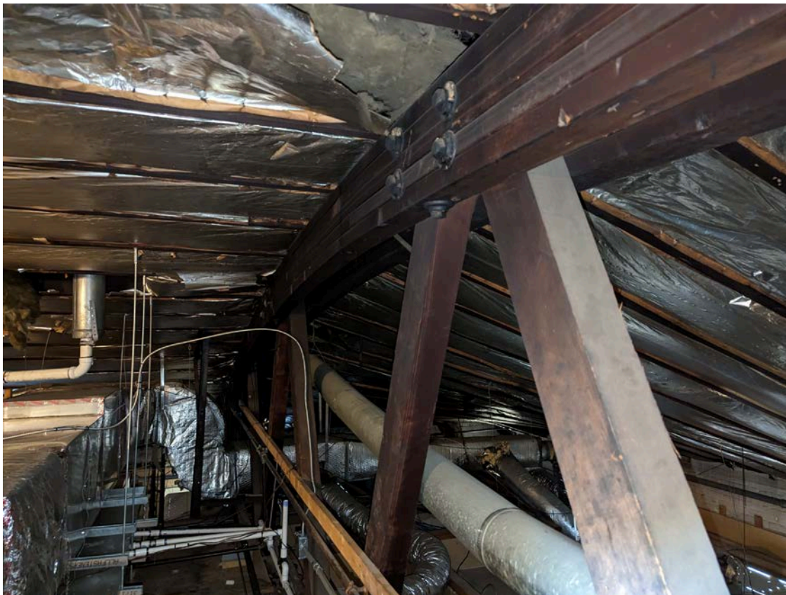
Photo #17 – Rear Roof – Bowstring Truss & Rafters above.
