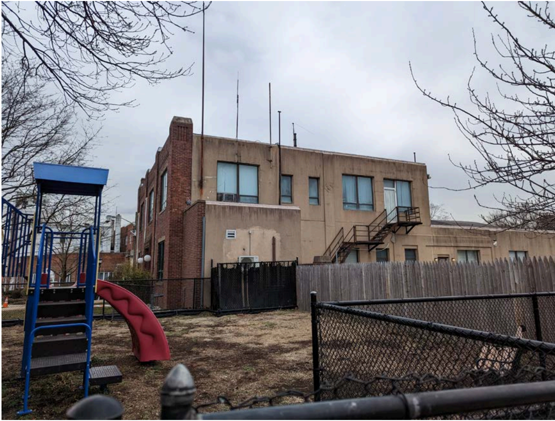
Photo #3 – Southwest View of Building.
