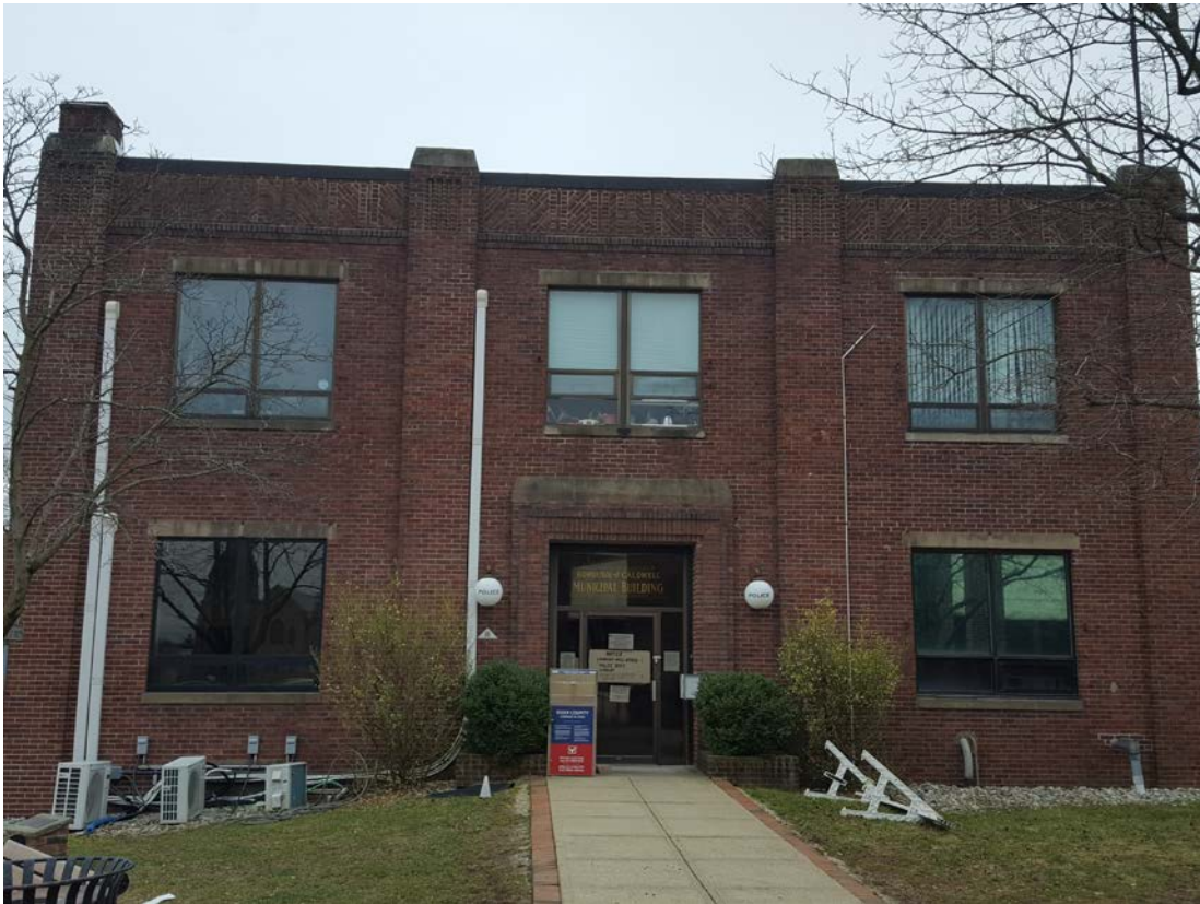
Photo #2 – Front of Building.
