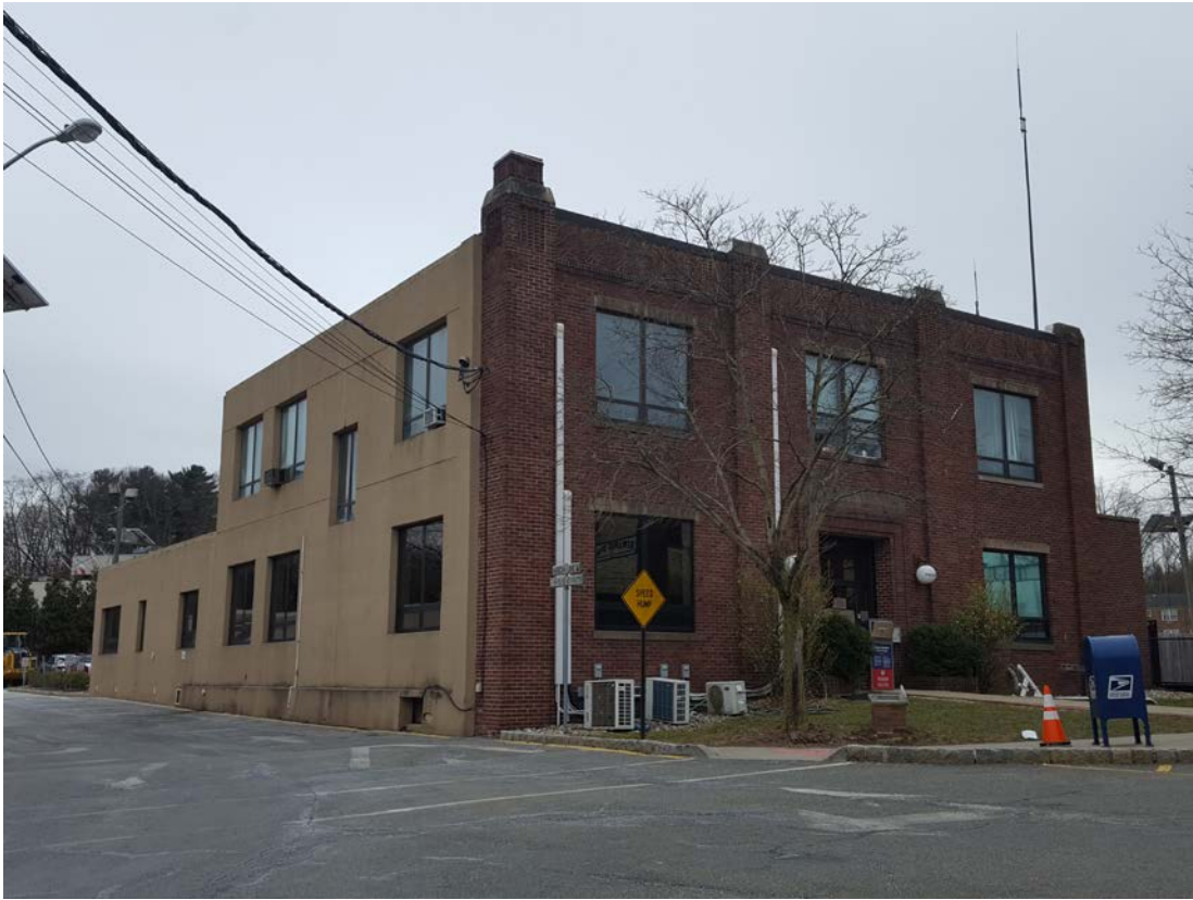
Photo #1 – Exterior Northwest Side of the Building.
