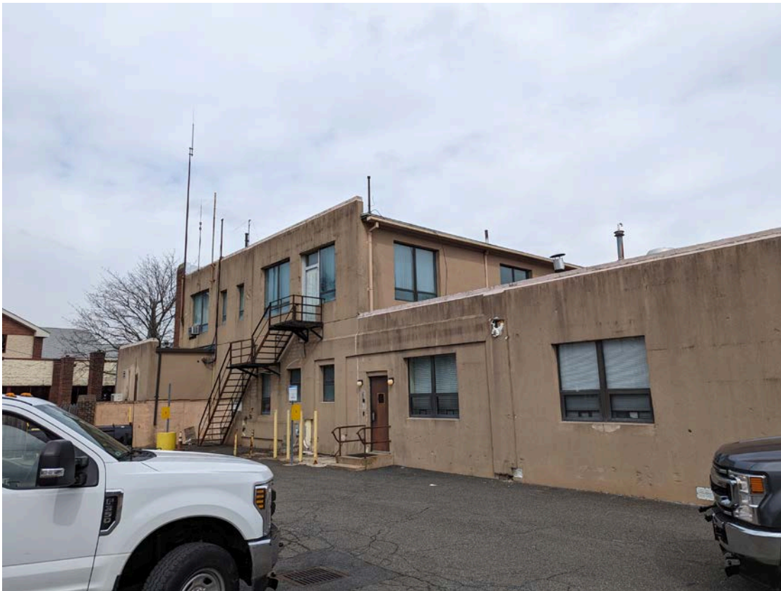
Photo #4 – South View of Building.
