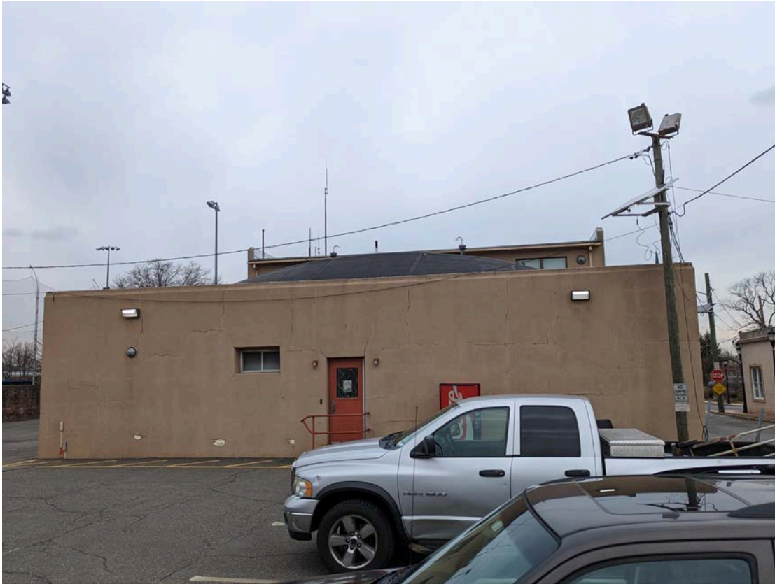
Photo #5 – East Side of Building.
