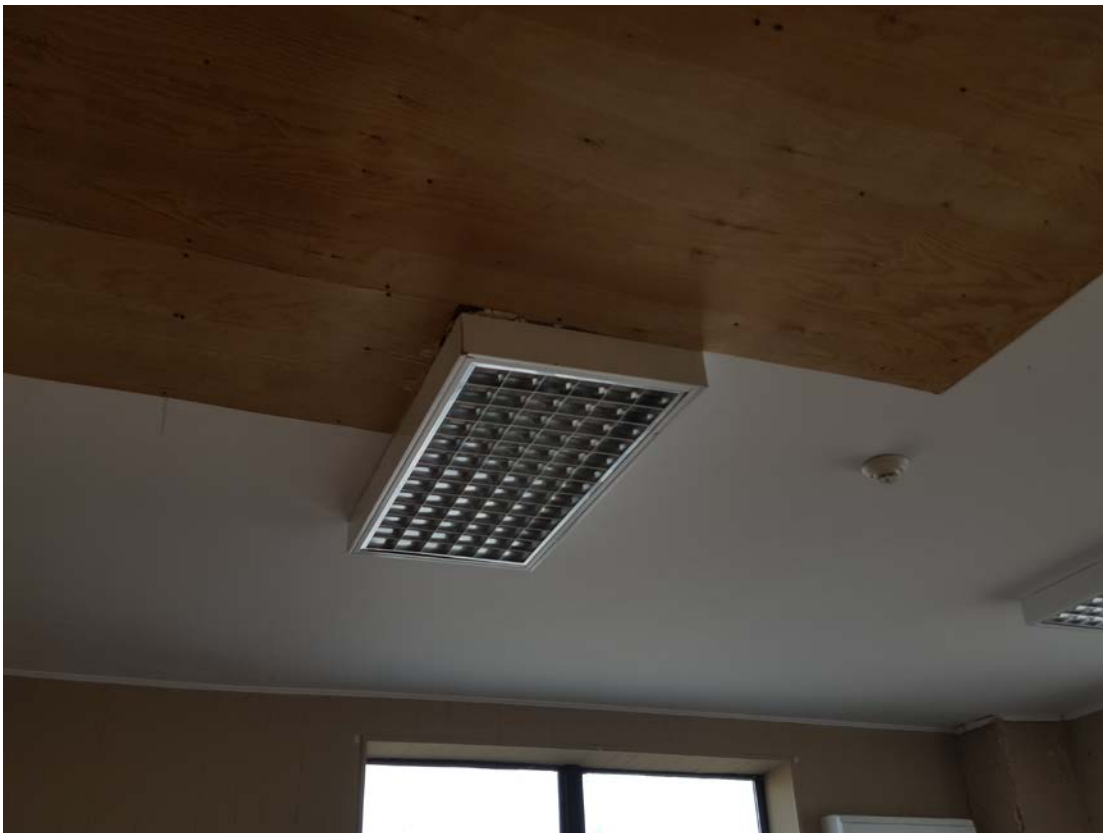
Photo #14 – Temporary Ceiling Repairs.
