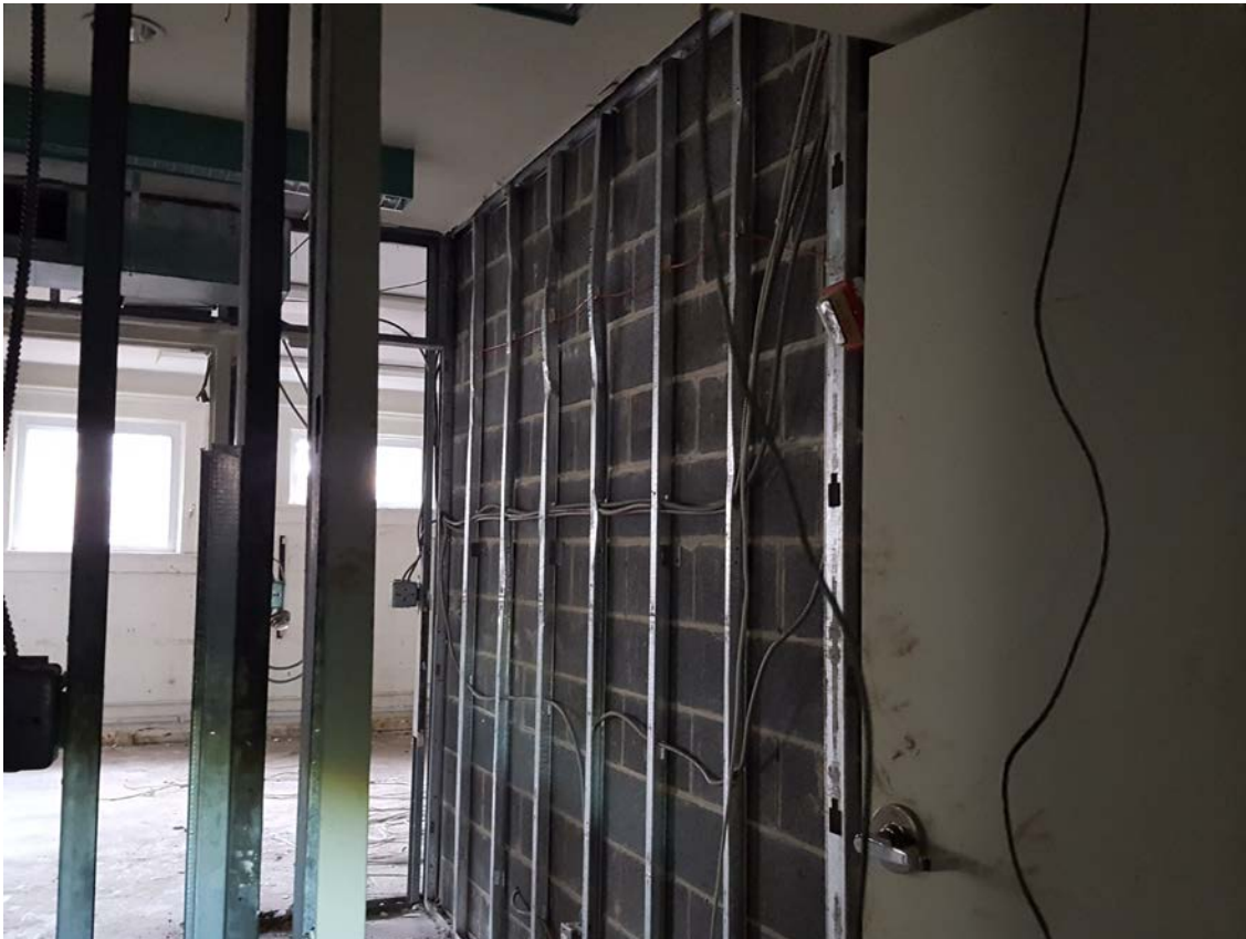
Photo #28 – Newer CMU Wall Near Entry of Original Building.
