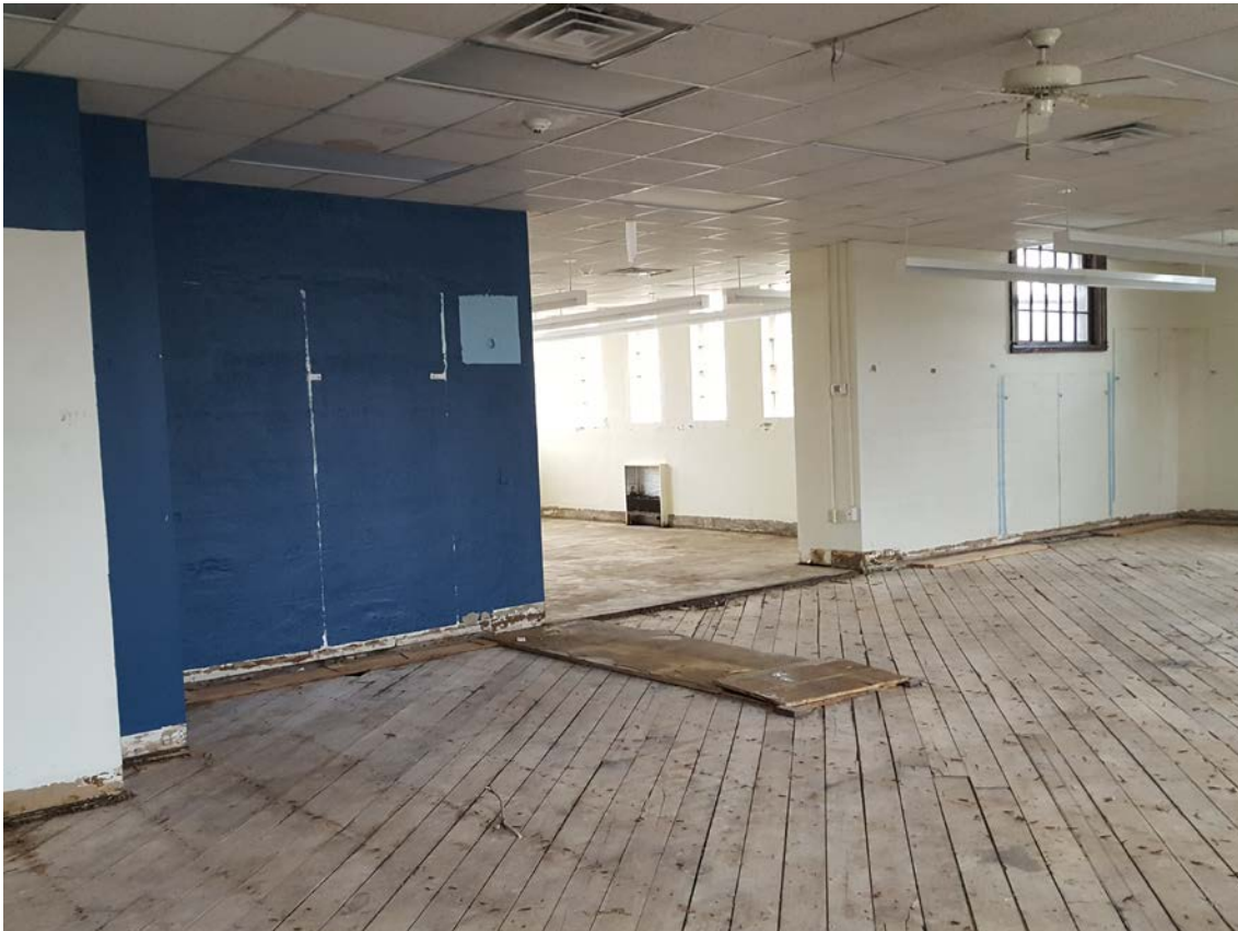
Photo #14 – Interior View of Space, Looking towards South Addition.
