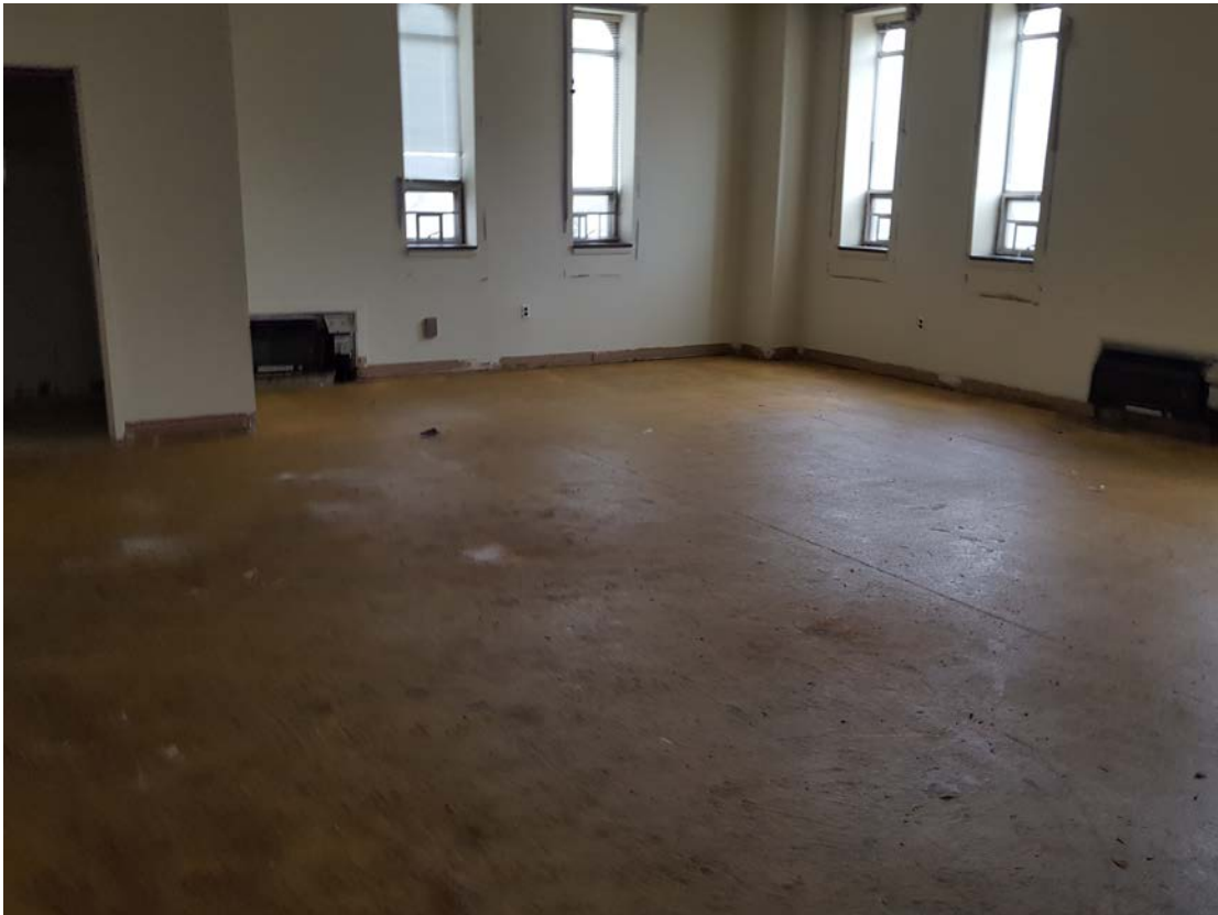
Photo #18 – Rear Addition Space – First Floor.
