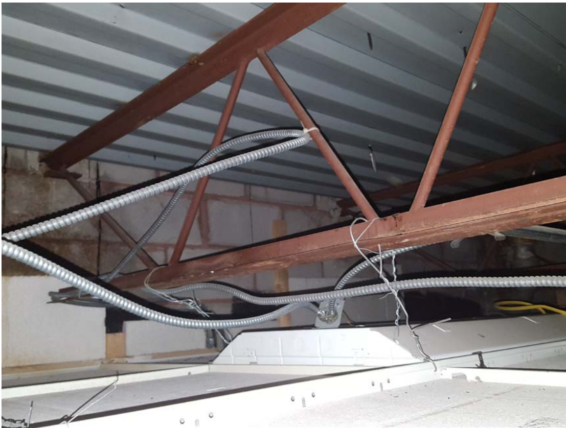
Photo #24 – Typical Roof Construction at East Addition.
