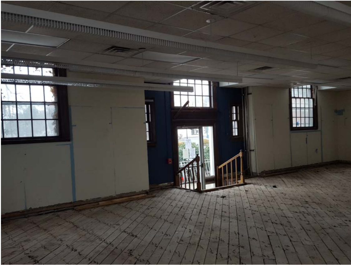
Photo #13 – Interior View of Main Entry – North Side.
