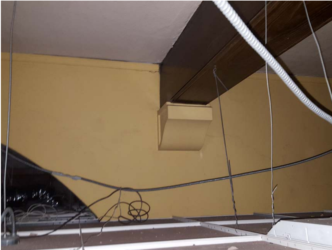
Photo #19 – Ceiling Cavity over Original Building – Dropped Beam 1 of 2.
