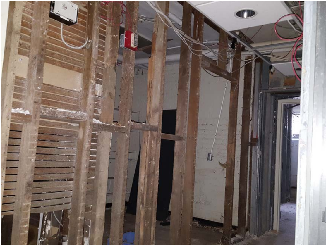
Photo #29 – Wood Bearing Wall at Northeast Corner of Original Building.
