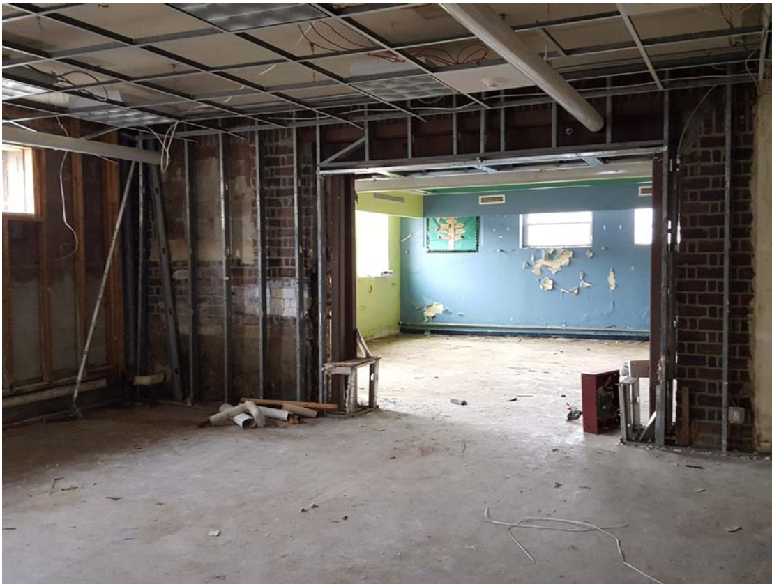
Photo #26 – Basement Level – Looking Southwest.
