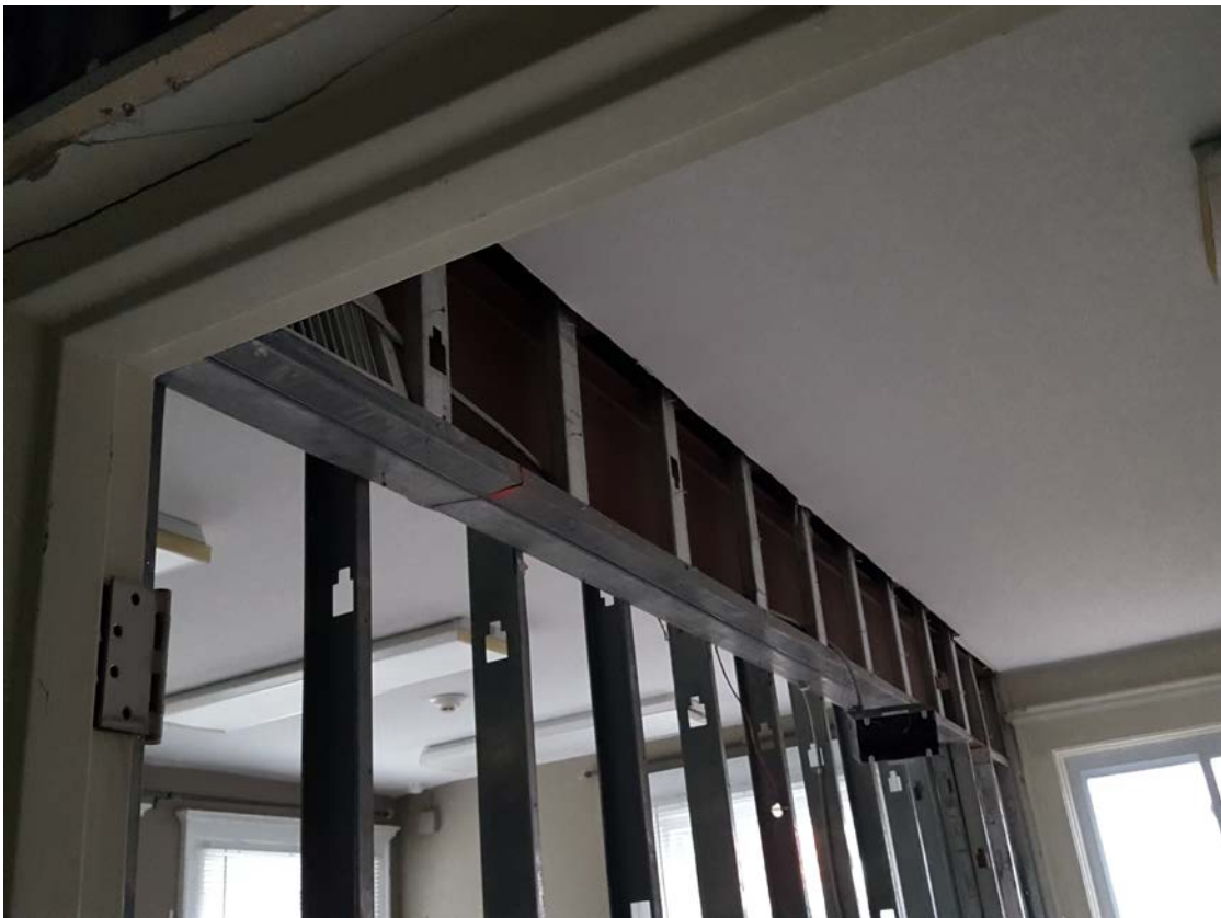
Photo #30 – Newer Steel Beam Supporting Wood Joists Above – Basement Northeast Section.
