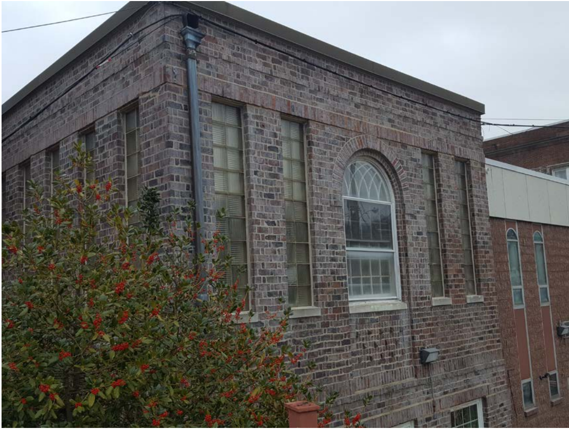
Photo #5 – Southwest View of Building.
