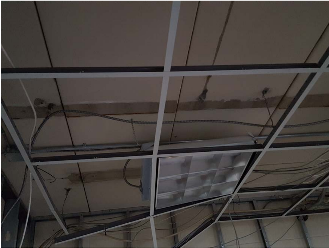
Photo #27 – Precast Concrete Plank at East Addition.
