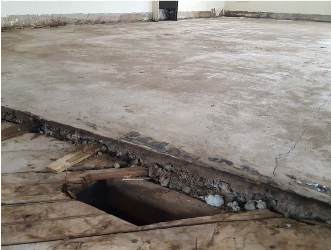
Photo #15 – Floor Transition from Original Structure to Addition.
